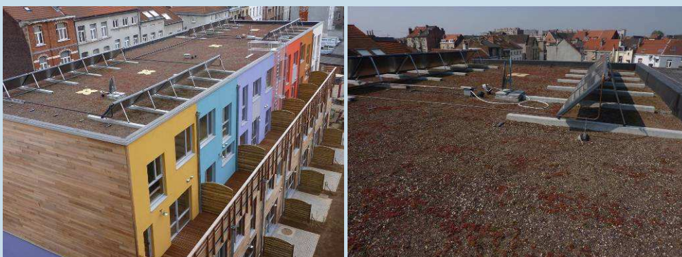
Figuur 1: groendak + zonneboiler (Bron: Architect D. Carnoy)
